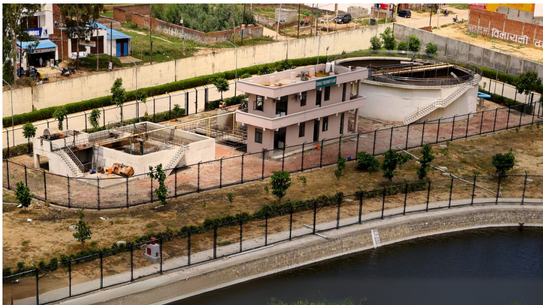
Sewage Treatment Plant
